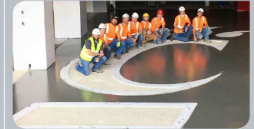
long-term strength and durability. Those characteristics were ideal for the University of Cincinnati arena floor.
