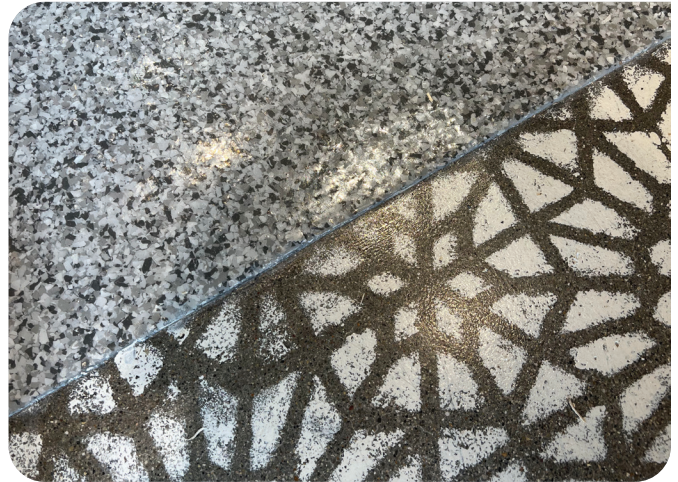
According to Hardig’s Kevin Kipp, the polished part of the job “was really creative.” The resinous flooring went in the kitchens of the 14 or 15 eateries and the polished went in the community areas.
