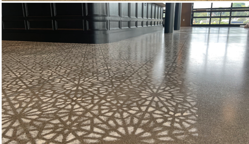
It took a 4- to 5-person crew from Hardig Industrial Services (depending on the task) to complete two different floor finishes at a new eatery in Ohio.
